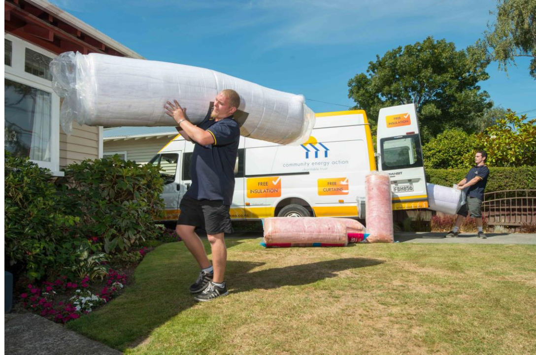
CEA Insulation Installer
